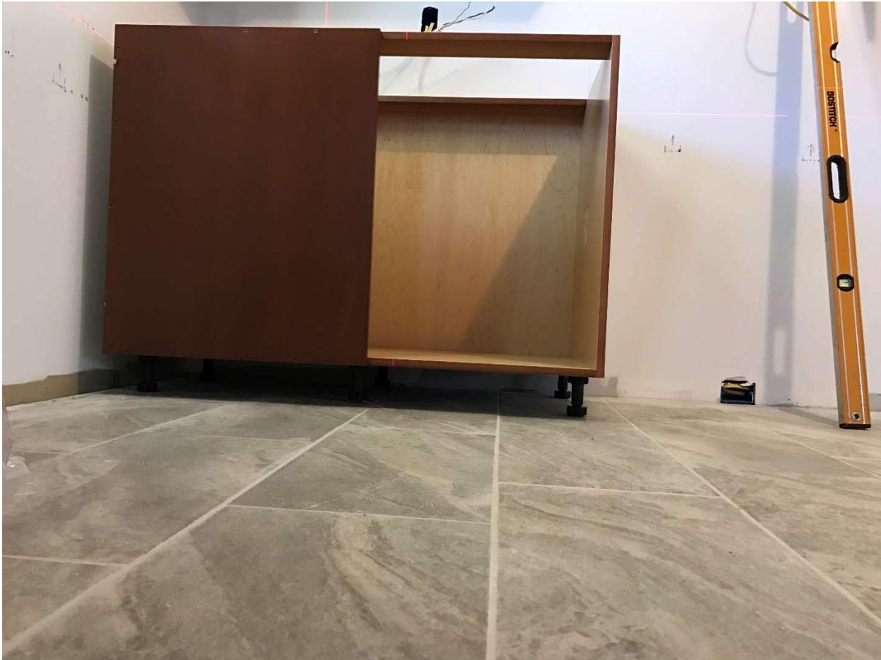
4. Screw cabinets to wall through 3/4" thick back at every stud using [3" PoweHead screws](#). Do not overtighten screw, pulling the cabinet out of level or plumb (you could shim the 10mm back scribe area if you need to).
