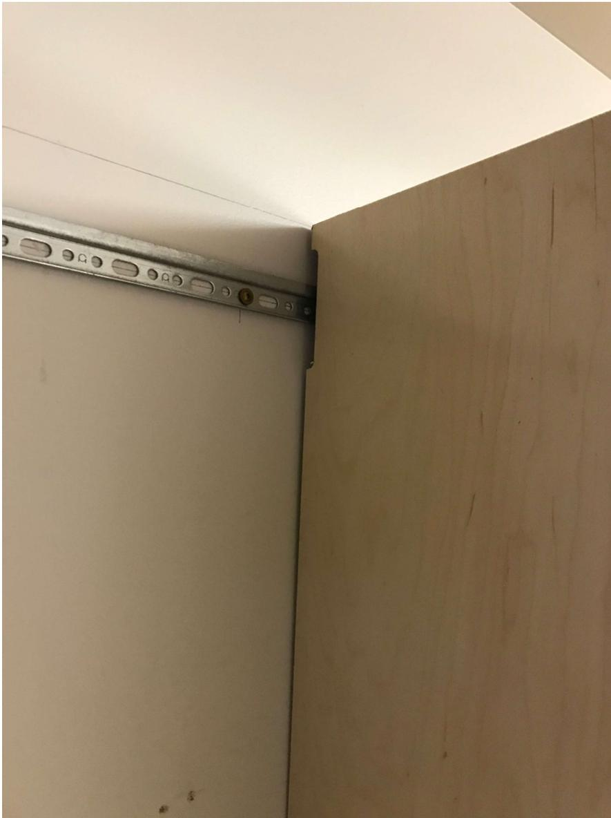
6. Clamp wall cabinets together with [quick clamps](#) and screw together with [1-1/4" screws](#).
