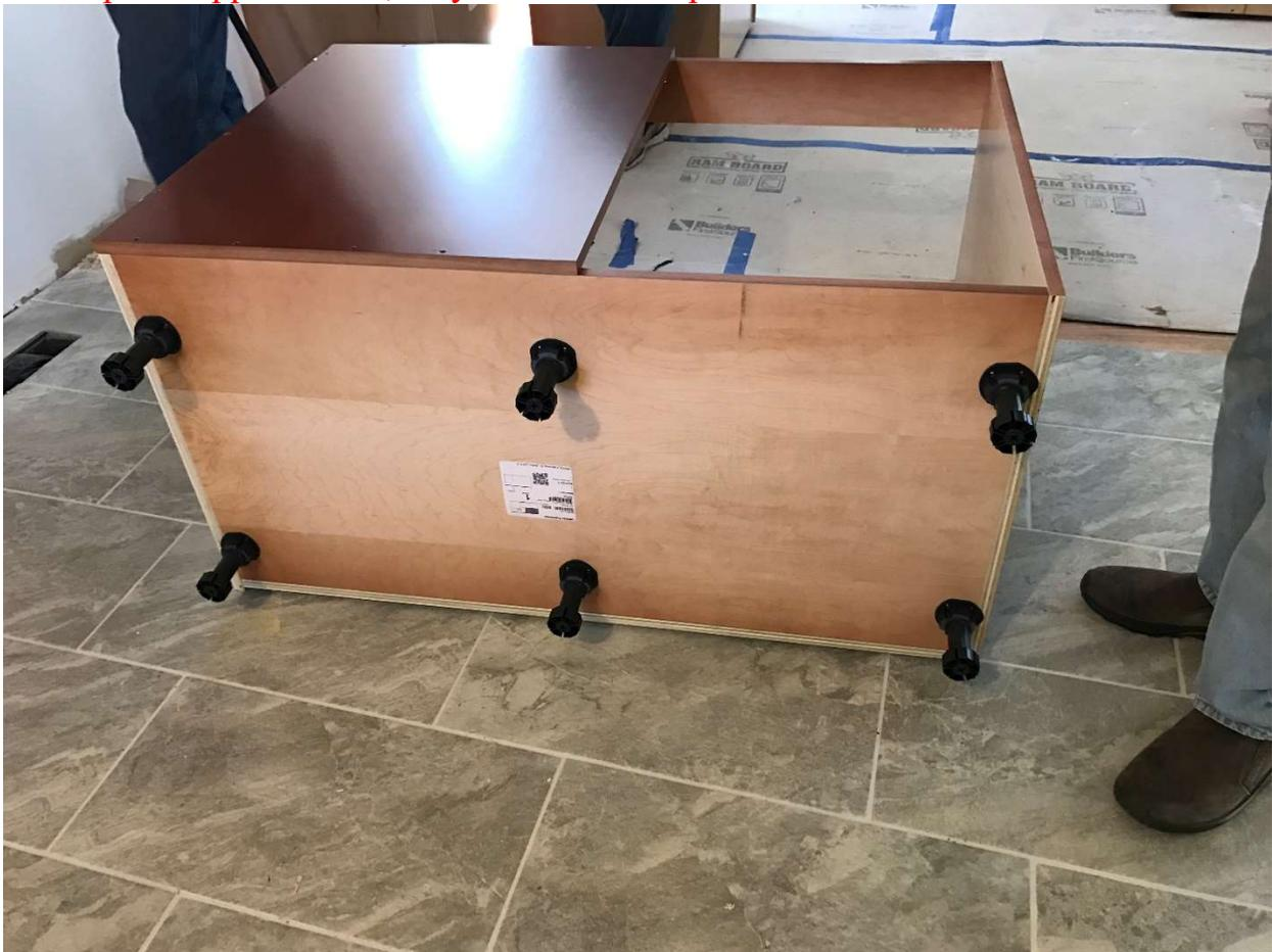
3. Start in corner and work out of corner putting cabinets in place and adjust back of cabinet up to level line on wall (you can use a [long flat head screwdriver](#) to adjust back legs using the slots in the foot of the leg), then plumb cabinet with front legs, clamp together with quick clamps and screw cabinets together using 1-1/4" screws .
